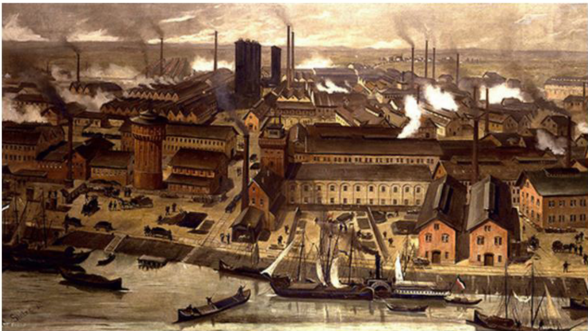
Image 3: Industrial plants on the Rhine river at Ludwigshafen. Source: “BASF Werk Ludwigshafen 1881,” by Robert Friedrich Stieler. Available in the Public Domain at https://en.wikipedia.org/wiki/File:BASF_Werk_Ludwigshafen_1881.JPG .
