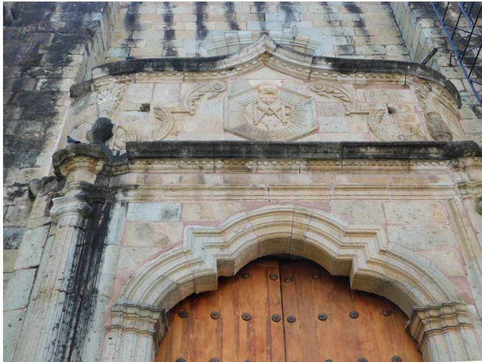
Image 4: Pointed/Ogee Arch in North Portal. Photograph by the Author.
