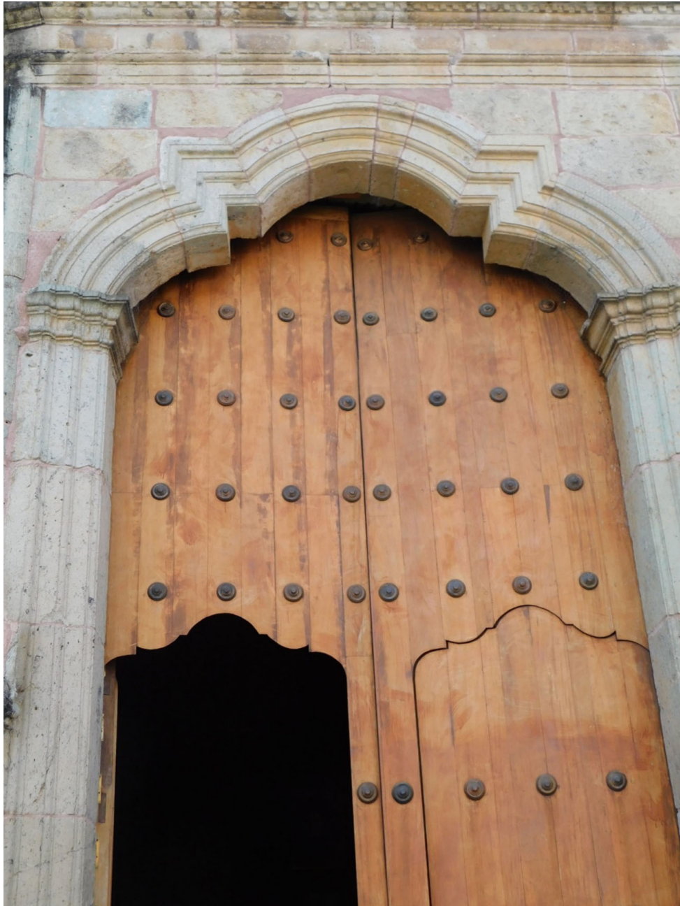
Image 8: Mixtilinear Arch - North Portal. Photograph by the Author.
